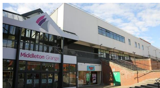
Middleton Grange Shopping Centre
